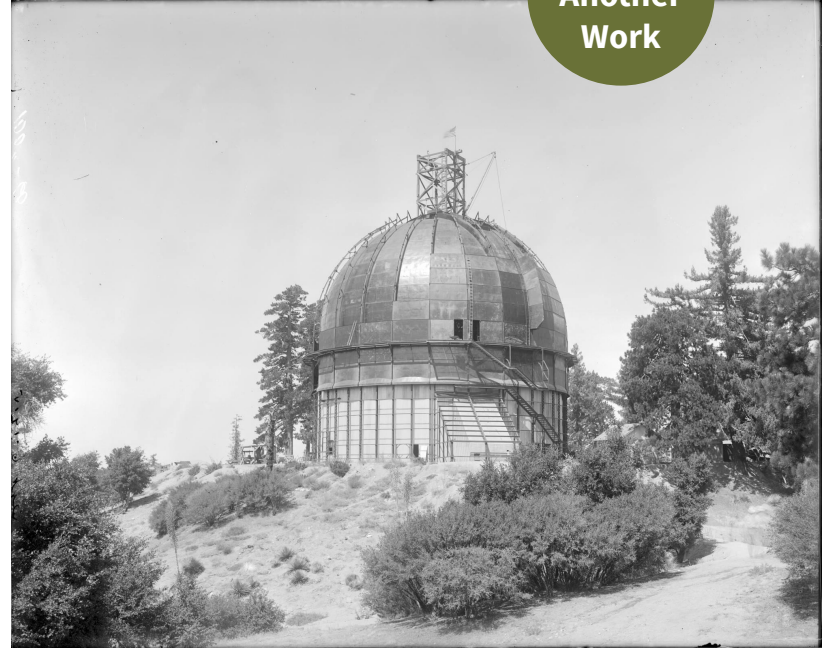
Partially completed construction of the 100-inch telescope dome of the Mount Wilson Observatory, 1915. The Observatories of the Carnegie Institution for Science Collection at The Huntington Library, Art Museum, and Botanical Gardens.
